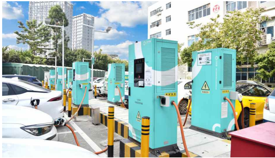
BYD Charging Project
