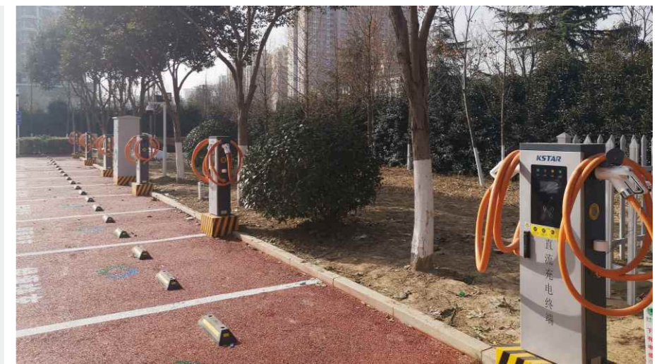
Shangqiu Municipal Project
