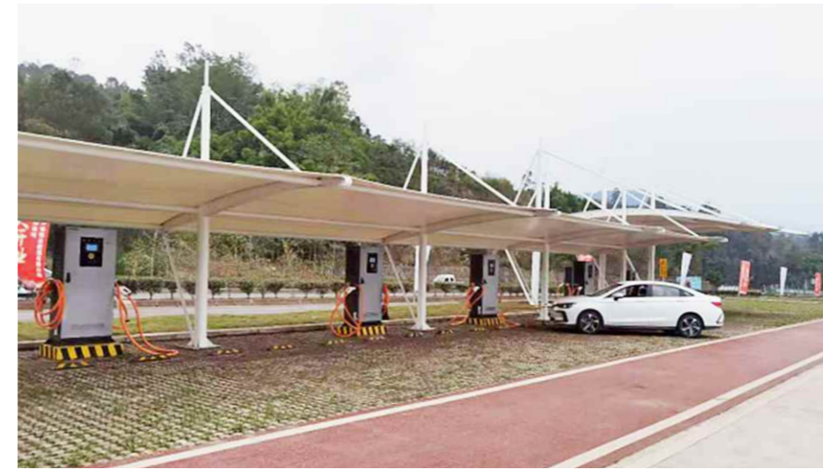
China Petroleum Project
