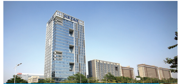
KSTAR Industrial Park at Guangming Industrial Zone, Shenzhen, China
