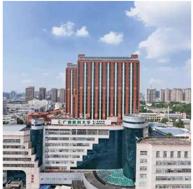
Guangxi Medical University Second Affiliated Hospital Project
