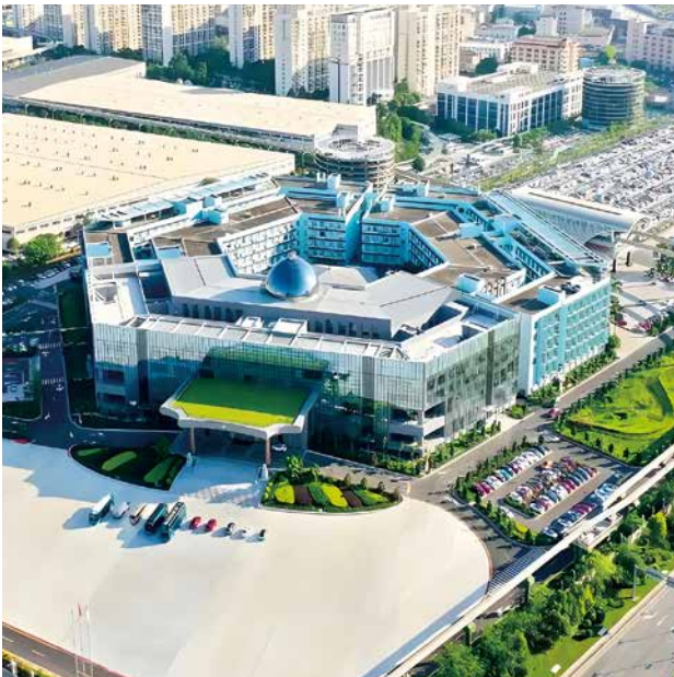
BYD Shenzhen&Shantou Plant 1 UPS Power Distribution Project
