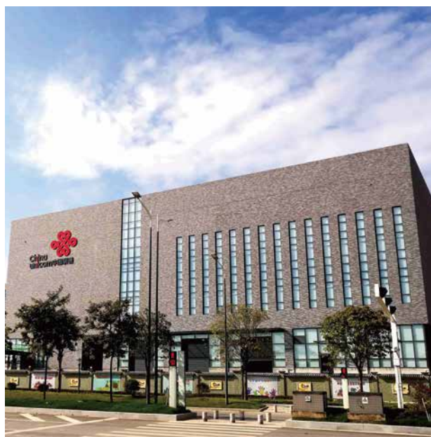
China Unicom Cloud Data Center Project
