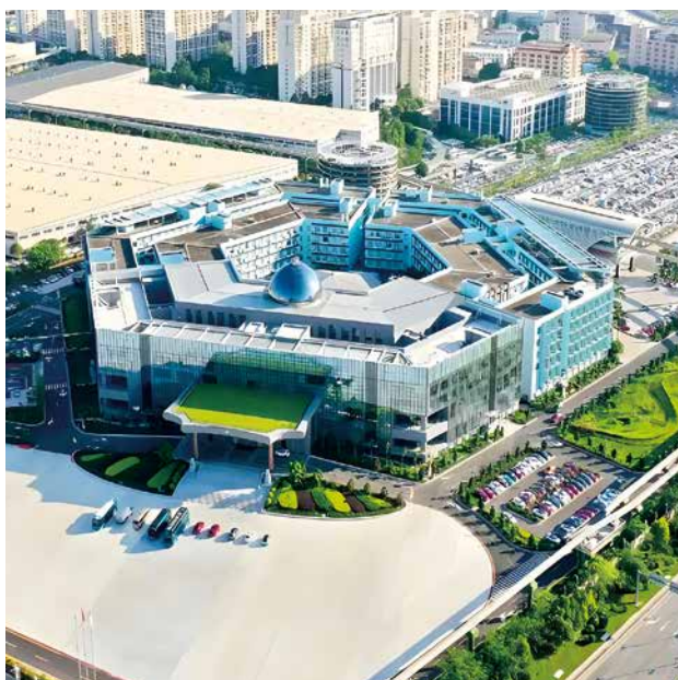
BYD Shenzhen&Shantou Plant 1 UPS Power Distribution Project
