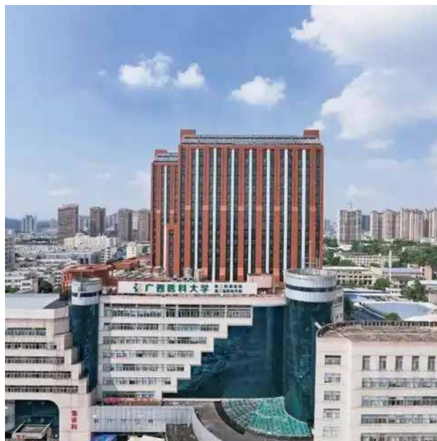
Guangxi Medical University Second Affiliated Hospital Project
