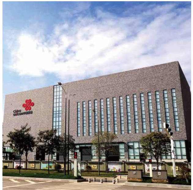
China Unicom Cloud Data Center Project
