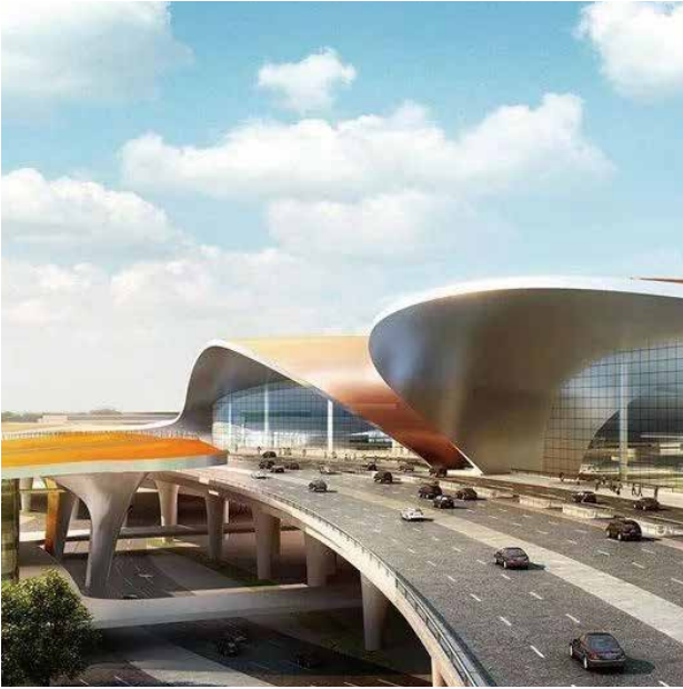
Beijing New Airport Eastern Airlines Base Project
