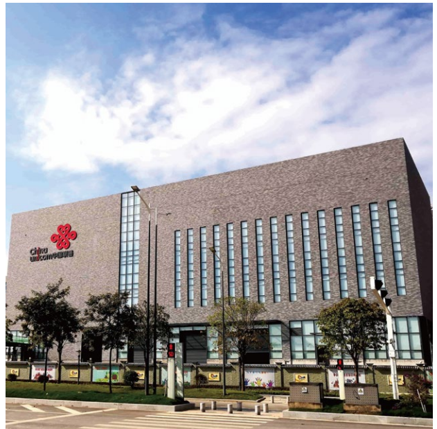
China Unicom Cloud Data Center Project
