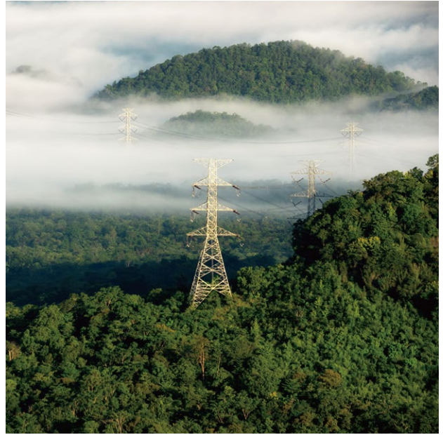
State Grid Project
