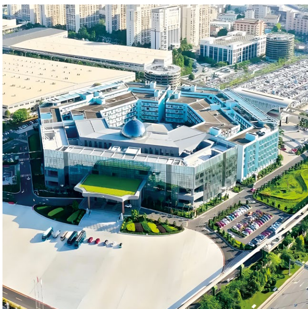
BYD Shenzhen&Shantou Plant 1 UPS Power Distribution Project
