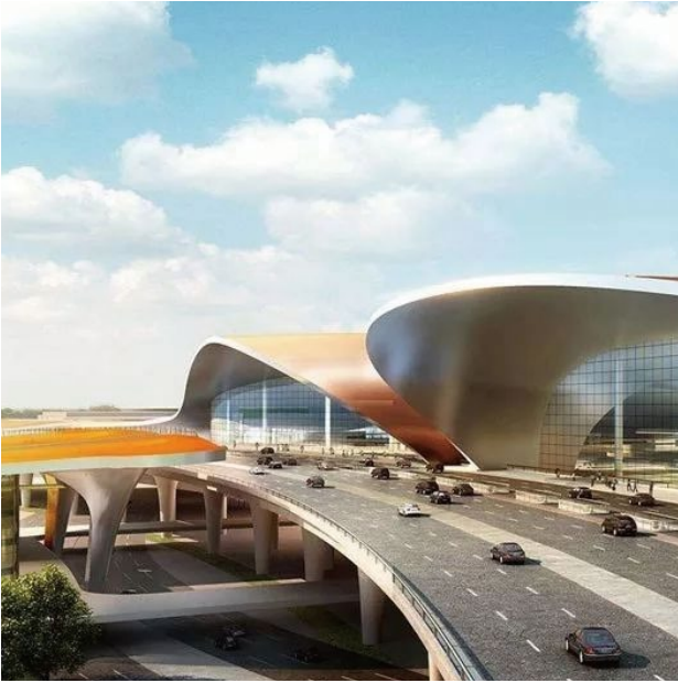
Beijing New Airport Eastern Airlines Base Project
