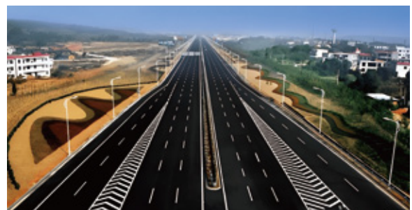
Ruili to Menglian Expressway Electromechanical Project
