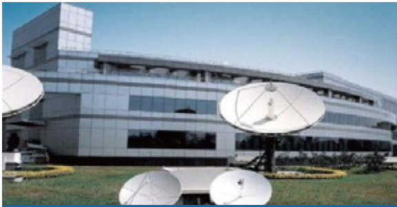
Shanghai Securities Waigaoqiao Earth Station
