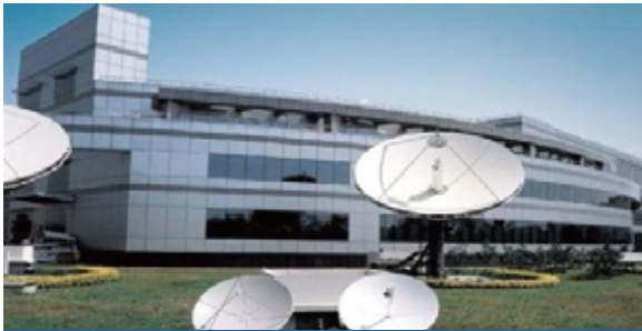
Shanghai Securities Waigaoqiao Earth Station
