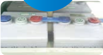
Leakage from battery cover
