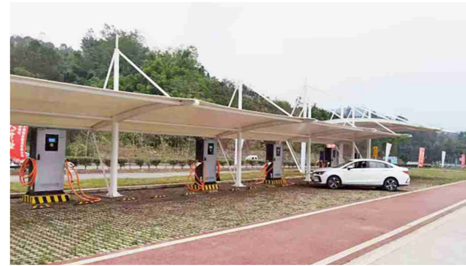
China Petroleum Project
