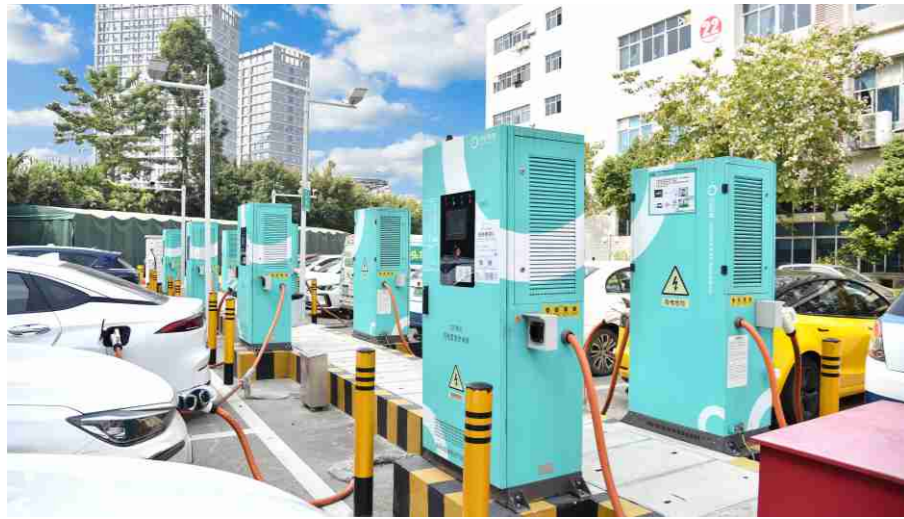
BYD Charging Project
