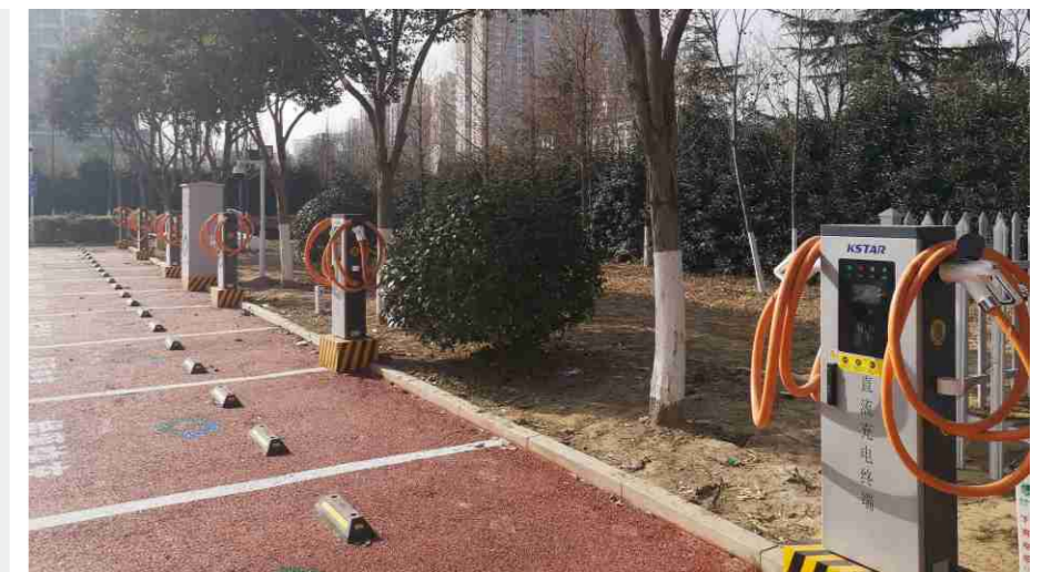
Shangqiu Municipal Project
