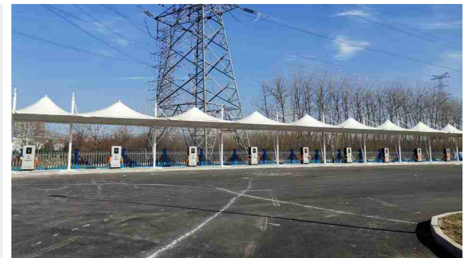
China Tower Project
